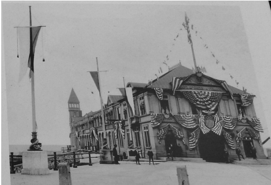
Pier A between 1909 – 1904, Lower Manhattan, within Battery Park 51
